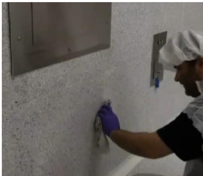
Photo #4: Remove excess caulking compound
