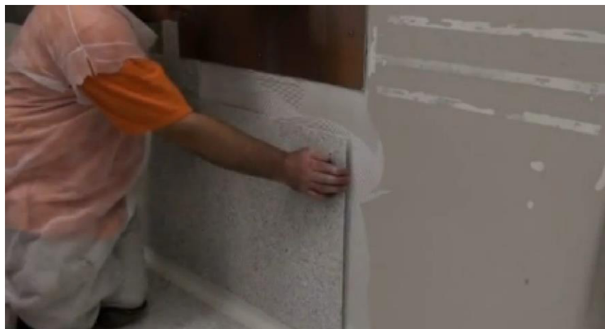
Photo #1: Placing tile into adhesive on wall.
