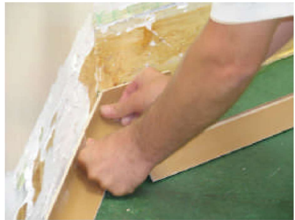
Photo #2: Secure base with adhesive
