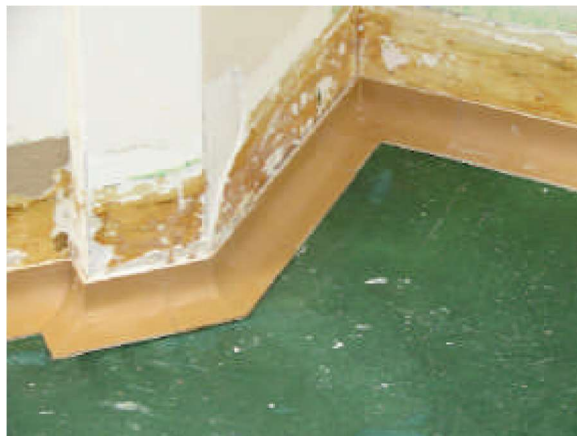
Photo #3: Finished sanitary base
