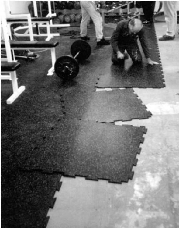
Four-Side Interlock Loose Lay Installation
