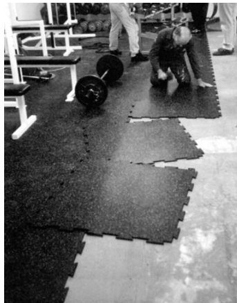
Four-Side Interlock Loose Lay Installation
