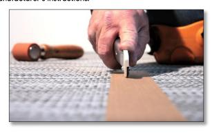
Cut the masking tape with a utility knife along the cut in the flooring. Shake the tube of cold-welding liquid and insert the needle deep into the joint. Slide the needle along the seam while squeezing the tube to adjust the flow. Let dry at least 30 minutes and remove the masking tape.
