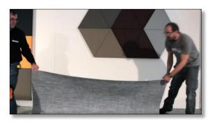
Let the adhesive dry according to the manufacturer's instructions and the type of adhesion (wet or dry adhesion). Once the adhesive is ready, lower the lifted half of the Fitnice® to the floor surface. Then lift the other half of the sheet and apply adhesive to the floor under it. Spread the adhesive carefully in the middle zone under the fold where the Fitnice® has been lifted.
