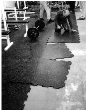
Four-Side Interlock Loose Lay Installation
