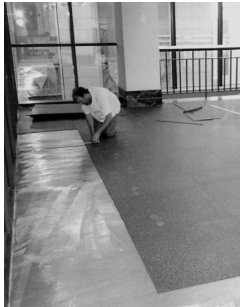
Square Cut Glue Down Installation
