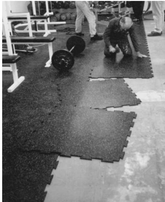
Four-Side Interlock Loose Lay Installation
