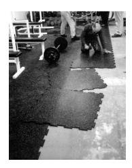
Four-Side Interlock Loose Lay Installation
