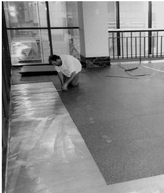
Square Cut Glue Down Installation
