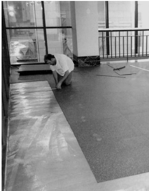
Square Cut Glue Down Installation
