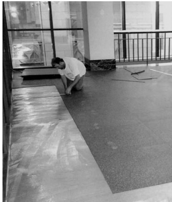
Square Cut Glue Down Installation
